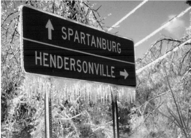
FIGURE C10-1 Glaze Ice Accretion Due to Freezing Rain.
